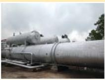
...thus the condensation tanks on each of the cylinders are eight feet in diameter by 140 feet long.
